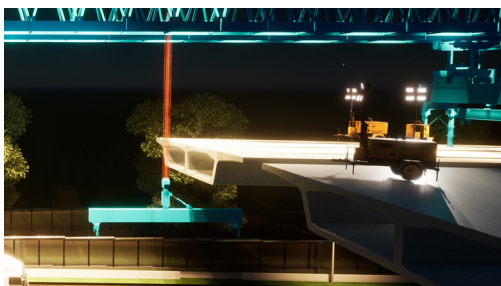
Fig. 9. Mitigation Measure Simulation based on Real-time Rendering Solution: A Case Study on Temporary Lights for Night Work
