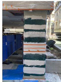
(b) Retrofit Method of Fiber Sheet
