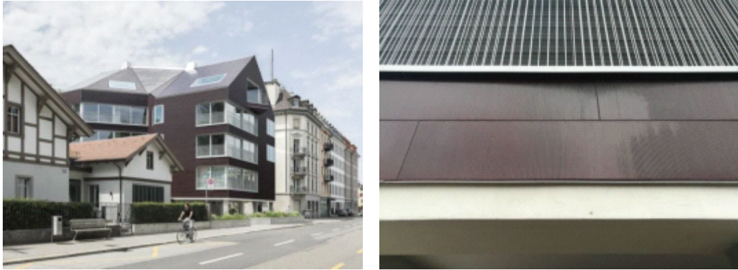
Digital ceramic print on glass/glass BIPV modules with various dimensions developed by ertex solar GmbH. Multi-family building Wohnhaus Solaris, Zurich (CH) (Source: HBF AG)
